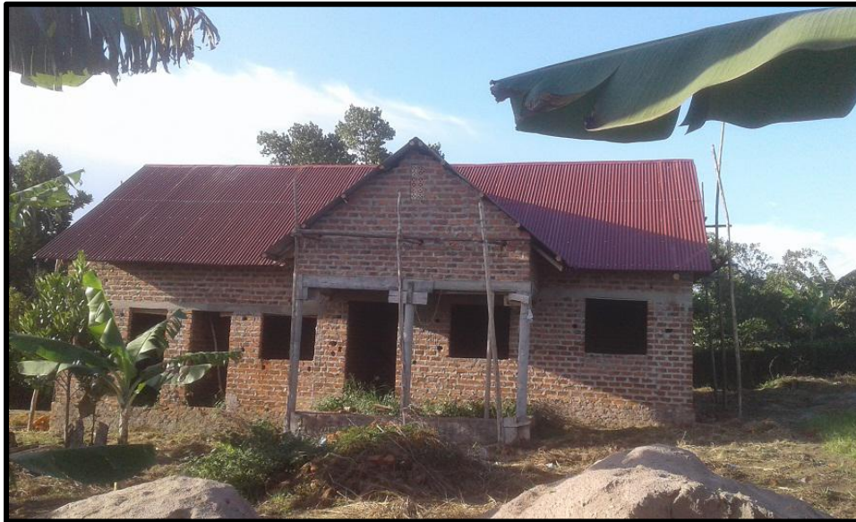
Construction progress of teacher's house.
