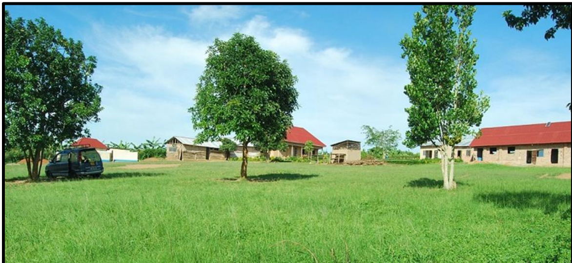
School view from bottom
